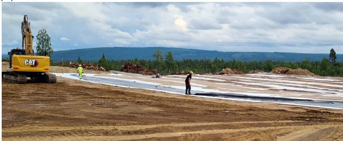
Figure 2 Vittangi Graphite Project trial mine groundworks during the period included lining of stockpile areas in preparation for commencement of excavations.
