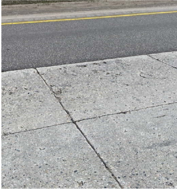
Figure 2 Mid-Section- Reference Slab -12 months Severe Surface Damage, Joint Rot, Pitting, Pop Outs
