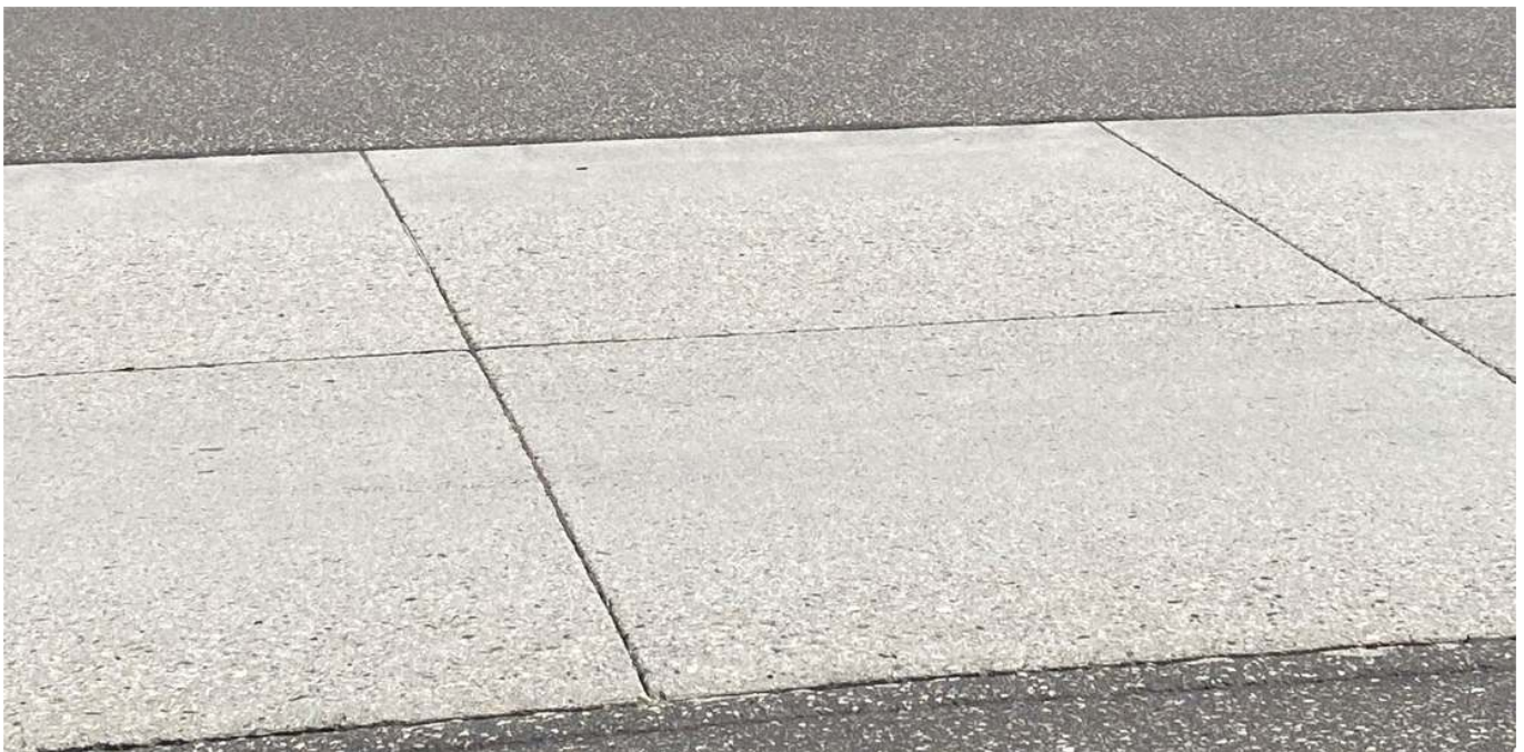
Figure 4 Mid-Section- EdenCrete® Slab – 12 months Top concrete surface partially worn off, No Scaling, No Surface Damage, No Pitting and Aggregate Pop Outs, No Rutting, No Joint Rot
