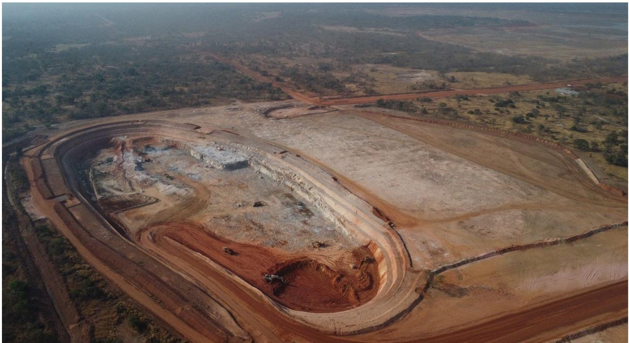
*Image 1 – Aerial view of Starter Pit and topsoil clearing of the next cutback*
