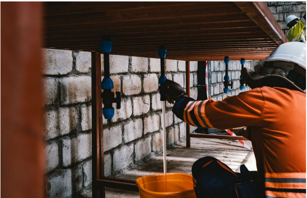
Figure 2: Water commissioning of desorption columns.
