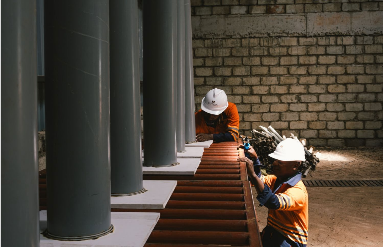
Figure 1: Inspection of constructed desorption columns.
