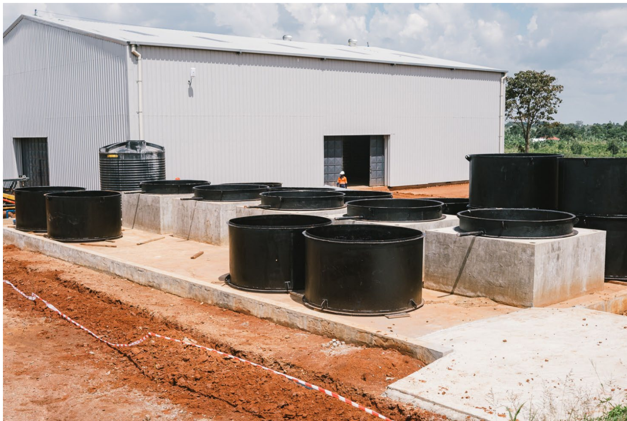
Figure 3: Crib shells which are being assembled for commissioning.
