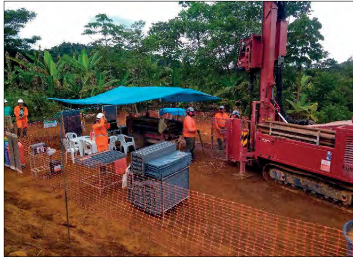
Figure 4. Sonic rig set up and safe drill site display. Gravel chips placed around rig working site prevent slippage.
