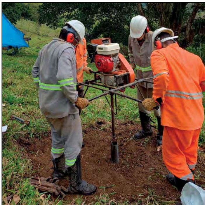
Figure 12. Mechanical auger in operation Source: BRE 2023
