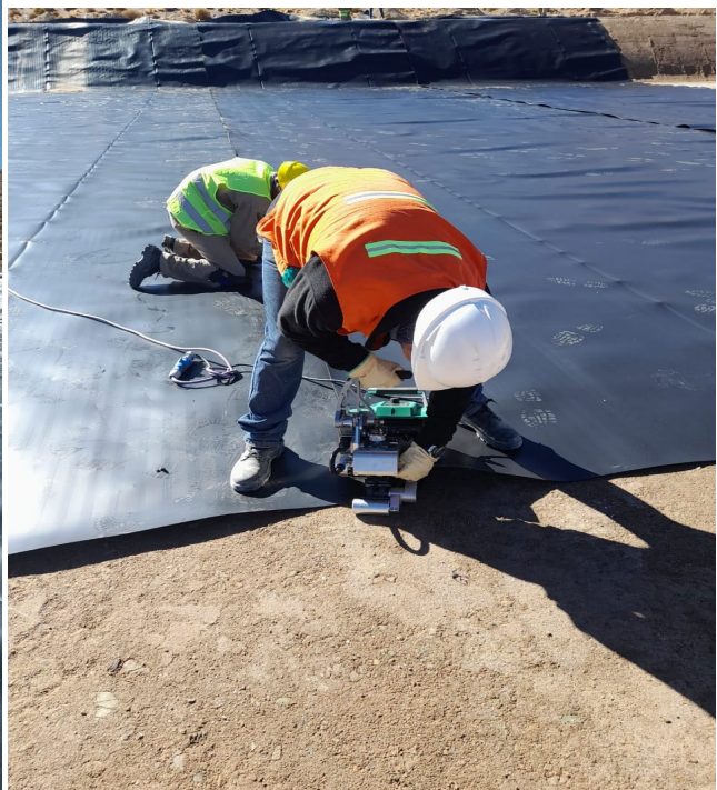
Figures 4 and 5 - Liner installation process Pond 1
