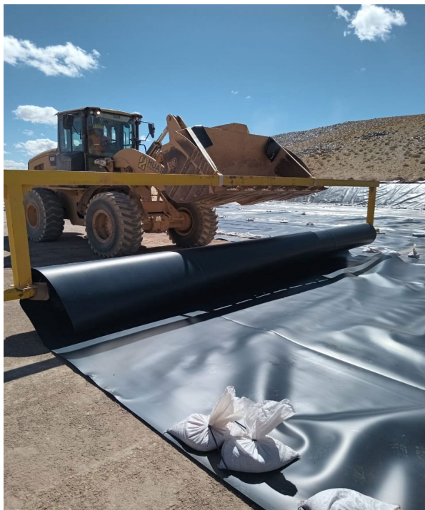
Figures 4 and 5 - Liner installation process Pond 1
