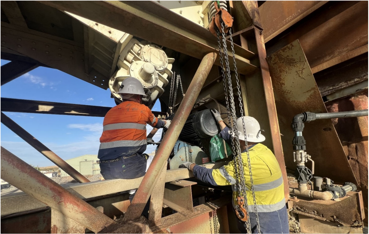
Figure 5: Black Cat maintenance team installing a replacement motor for primary crusher pan feeder.
