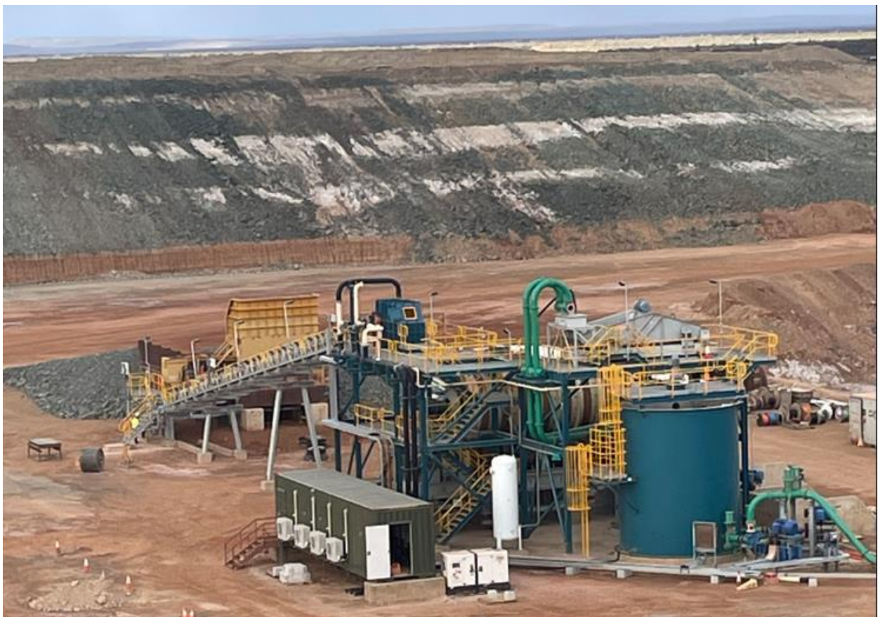
Figure 8-1: Wiltails feed system to CIL plant (TSF Western Cell in the background)
