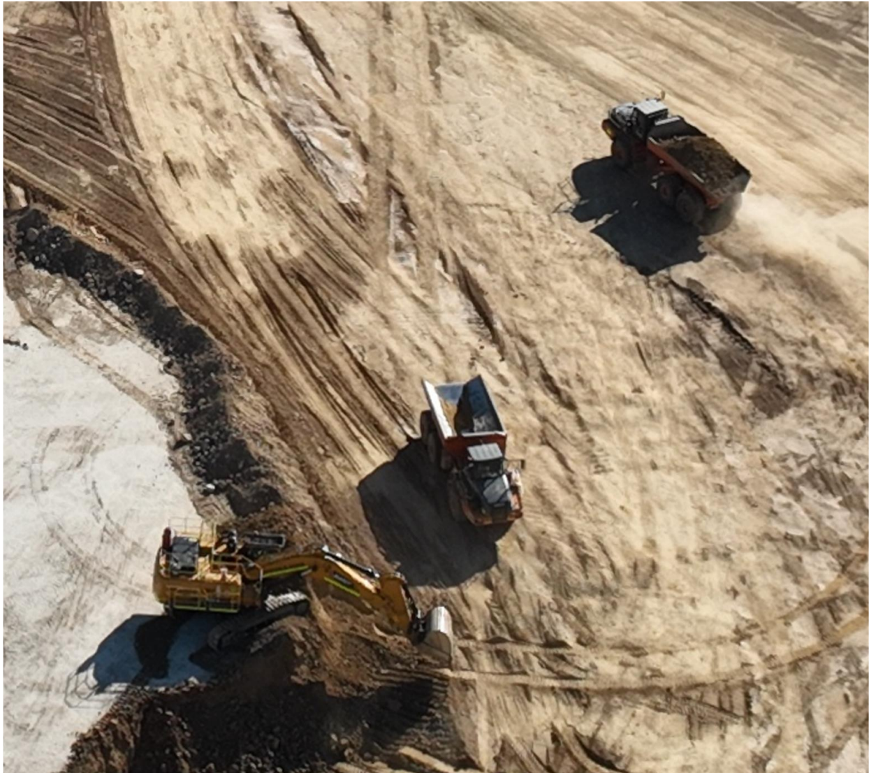
Figure 8-3: Wiltails - TSF Western Cell Tailings Reclamation – Excavator and Trucks
