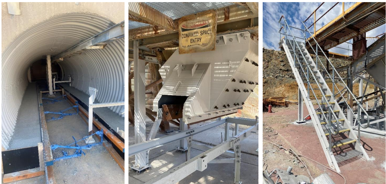
Figure 2: Mineral Hill plant - structural steel replacements and refurbished fine ore bin tunnels.
