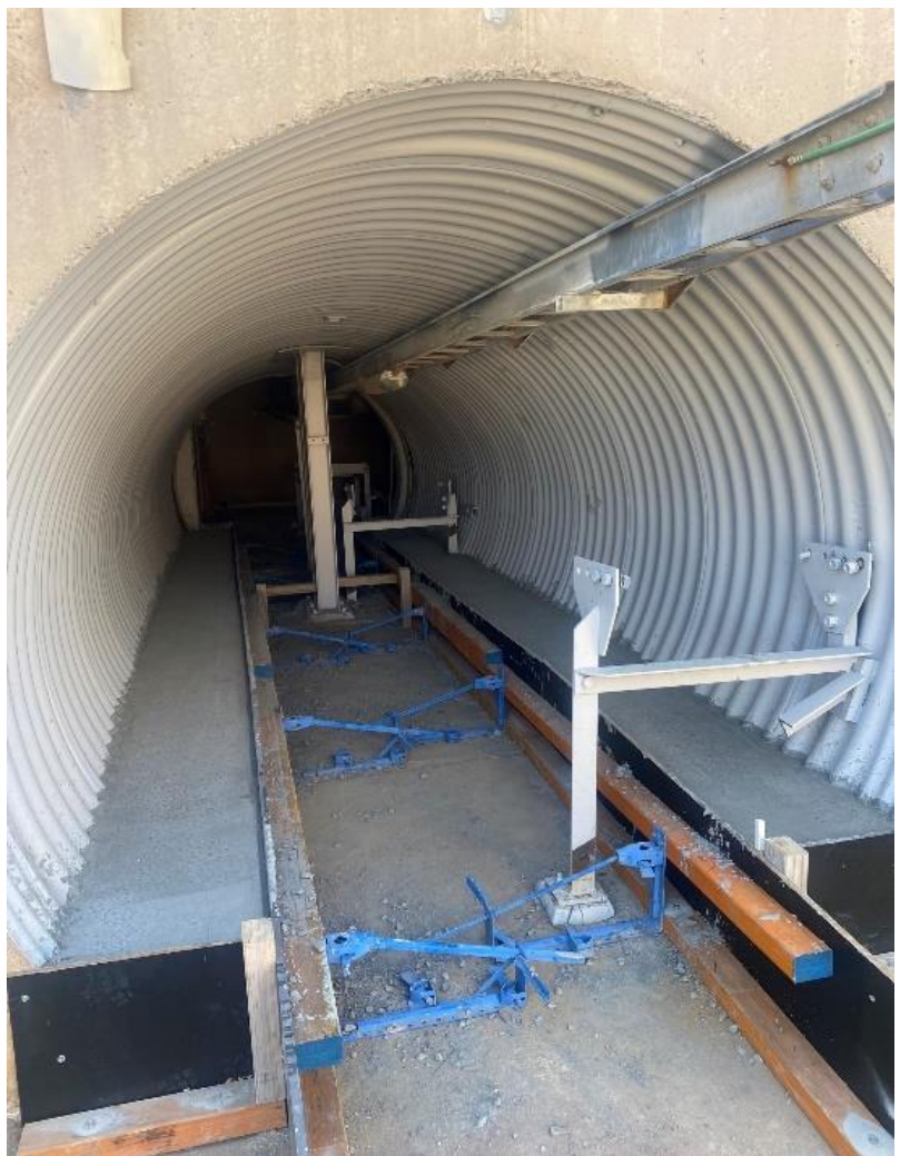
Figure 7: Refurbished conveyor tunnel from the fine ore bins up to the ball mills.
