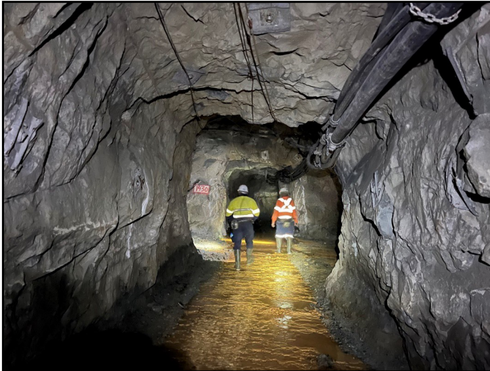
Figure 3. On-site workers in Amalgamated Adit/640L mine access point for the Reward gold mine to the Gold plant, with clean floors, good quality ground works and service pipes, all in very good condition
