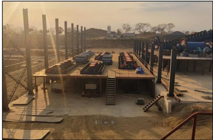
*Figure 2: Steel platforms around the grinding and flotation circuits within the Concentrator Building (left) and the start of the installation of the building steel framework (right).*
