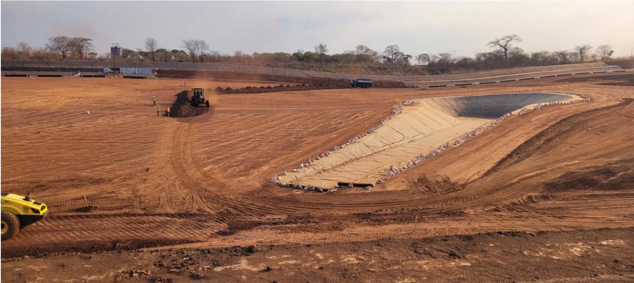
*Figure 5: Installation of drainage pipes and HPPE liner.*
