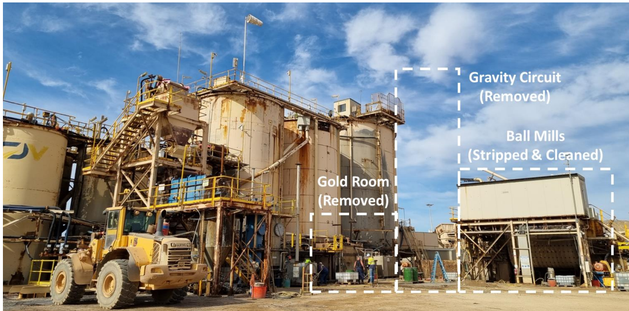
Fig. 6 – Central Gawler Mill with gravity circuit, gold room and other key equipment removed 7
