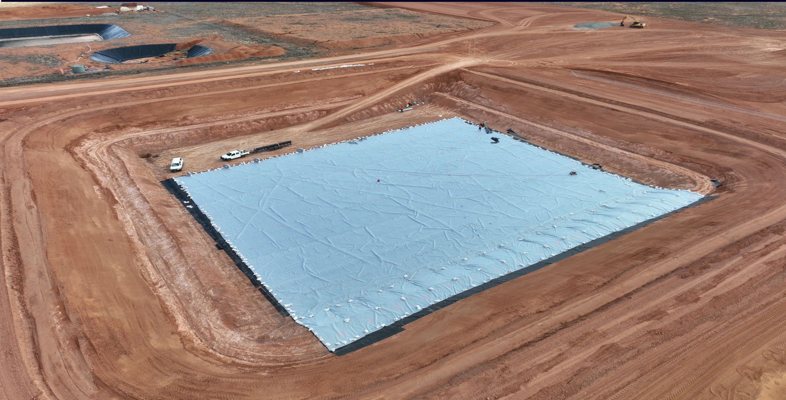
Gypsum pond lining being installed
