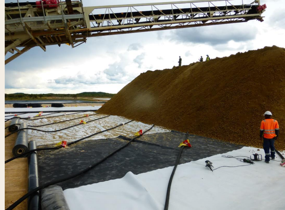
Figure: Example of Heap Leach construction
