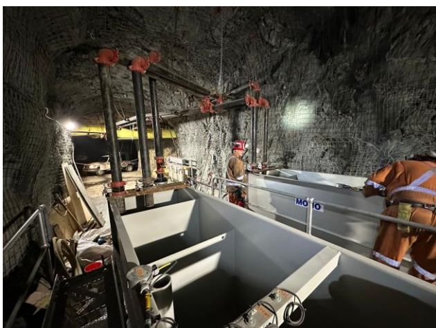
Figure 4: New Sugar Zone pump station installation, improving pumping capacity, reliability and reducing dewatering cost
