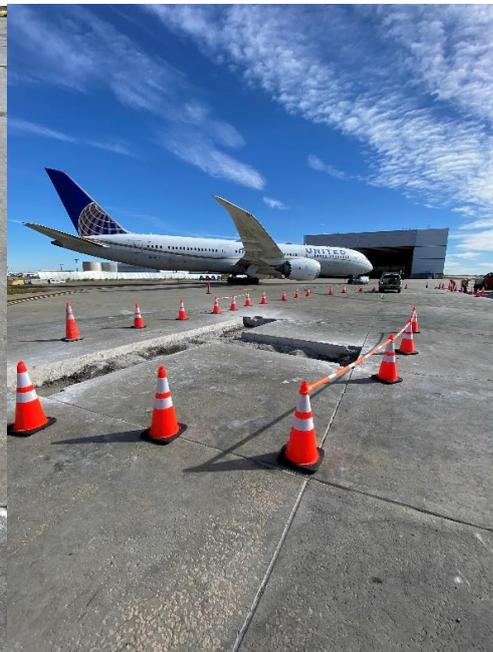
Figure 2. Concrete slabs being replaced
