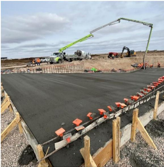
Figure 3. Longs Peak Dairy - fluid retention basin floor.
