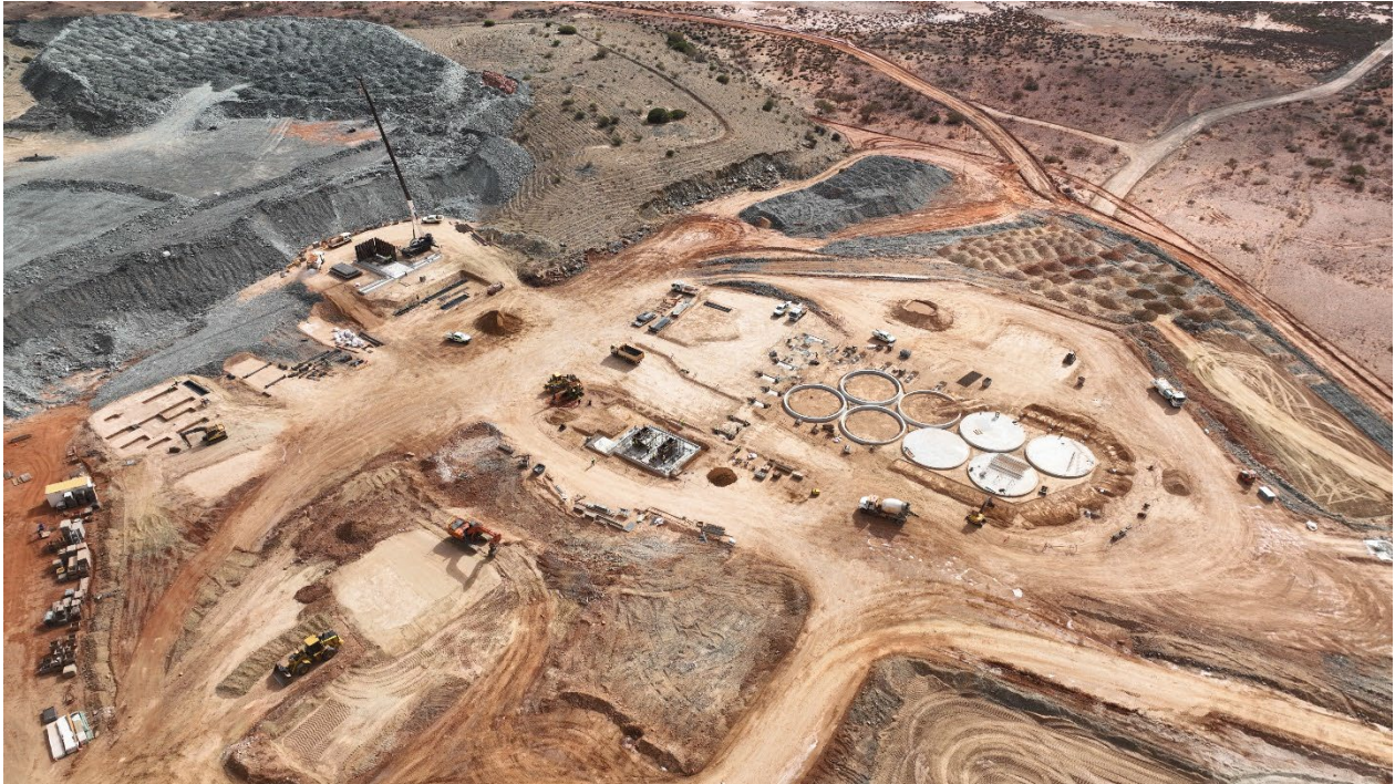
Figures 1-3: Top - Overview of processing plant works as of 15/11/2023, with critical path CIL ringbeams prominent in the centre. Bottom left - Closeup of mill raft concrete pour. Bottom right - completed CIL ringbeam concrete pours.
