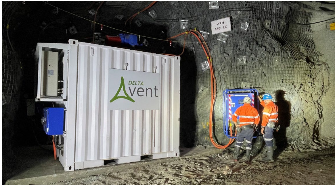
Figure 14: Delta smart vent allowing ventilation on demand installed at Bellevue, delivering a forecast 30% energy consumption savings and associated greenhouse gas emissions reductions
