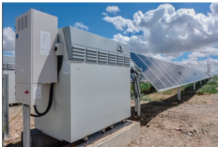
Figure 8 A Vanadium Redox Flow Battery powered by solar panels, ideal for homes, farms, towns, and suburbs
