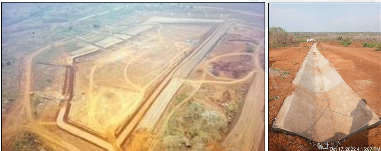
Figure 4: TSF construction progress (left) and the continuation of the minor concrete works through the construction of the stormwater drainage (right).
