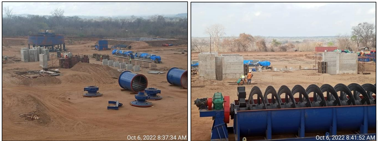
Figure 3: Concrete foundations for the rod, pebble mill and first bank of floatation cells (left) and the large spiral classifier with mill foundations (right). * Note the shells, bearings and ends of the rod and pebble mills laid out for assembly and installation.
