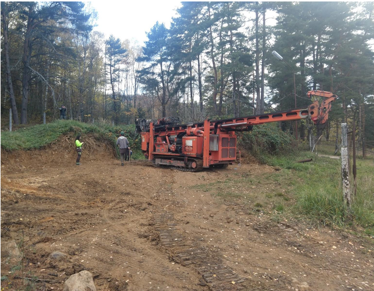
Figure 1: Diamond drill rig set up at the first target area, site preparation completed, location of drill hole SSD-01
