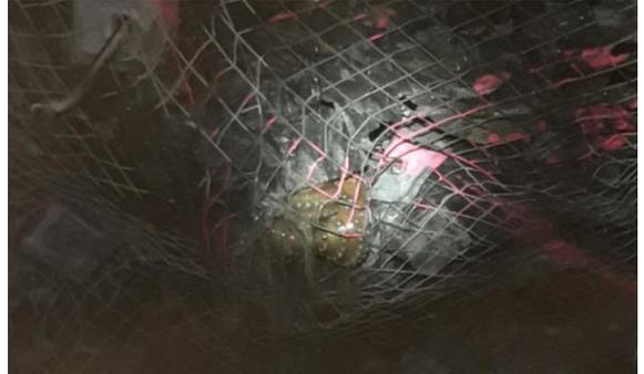
**Hoisting shaft Leg 1, raise-bore pilot-hole break-through on target at the mid-shaft access**
