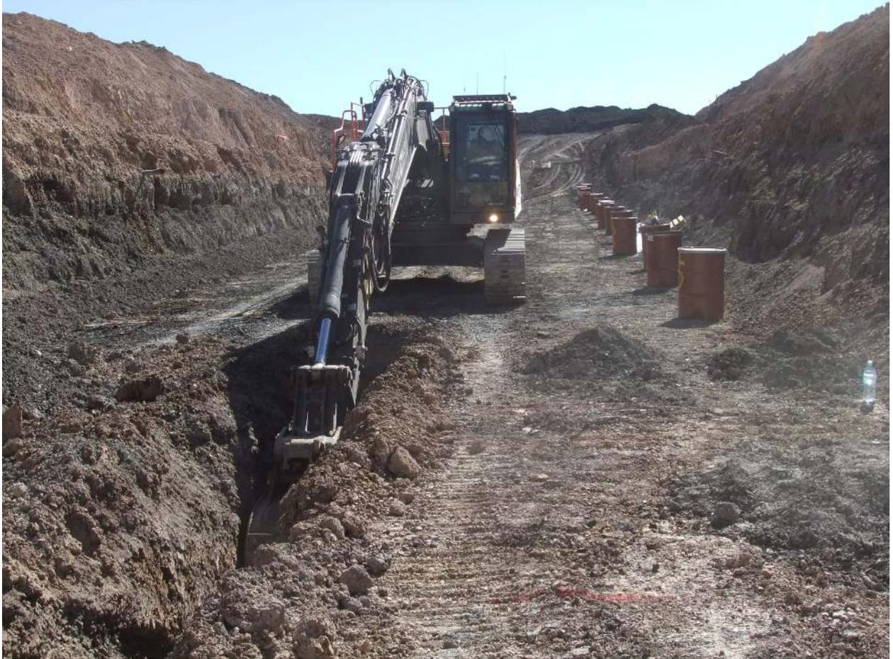
*Image 2 | Excavating sampling trench into the heap leach pads*
