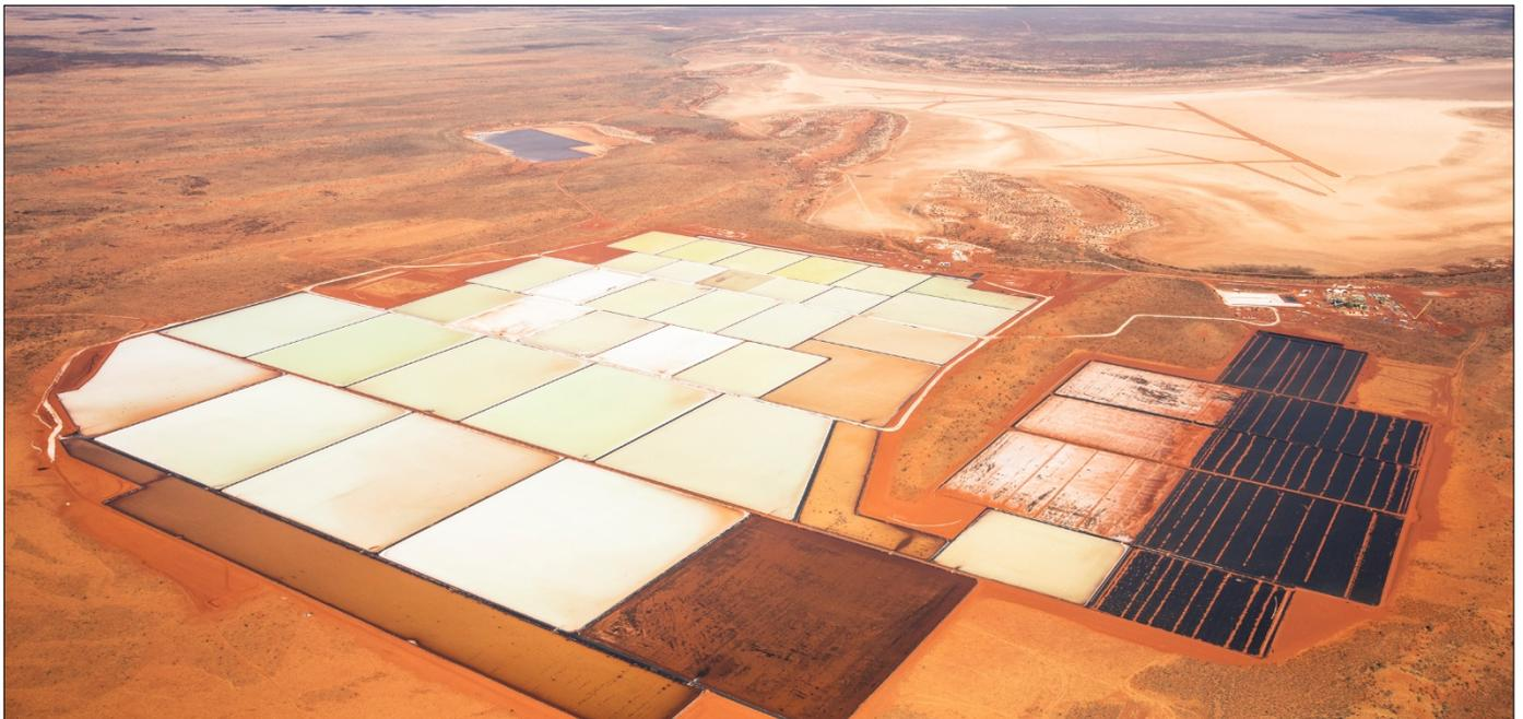
More than 2,400 rolls of HDPE liner were used to cover the laser levelled, tiered and graded area which, if rolled out end to end, would be approximately 500km long or the same as the straight-line distance from Sydney to Canberra and back. Completing this work required more than 3,000 man-days of effort across multiple contractors.
