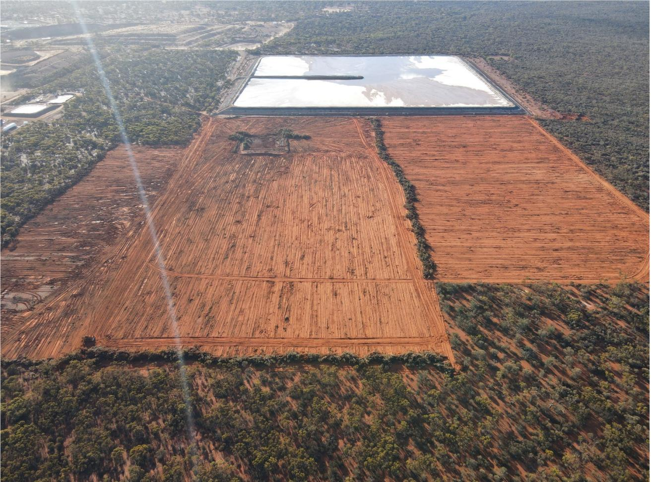
*Clearing & topsoil stripping for TSF Cell B construction at Davyhurst in progress*
