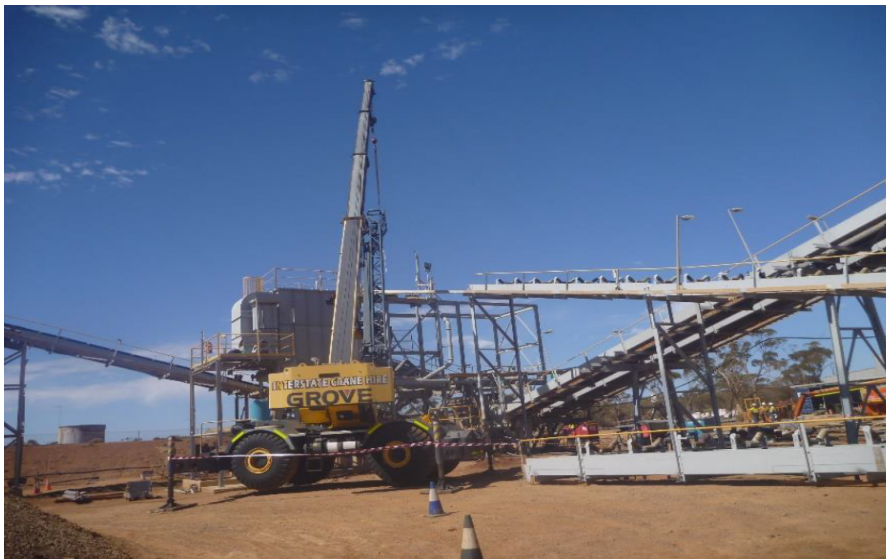
Upgrading conveyors to screening plant
