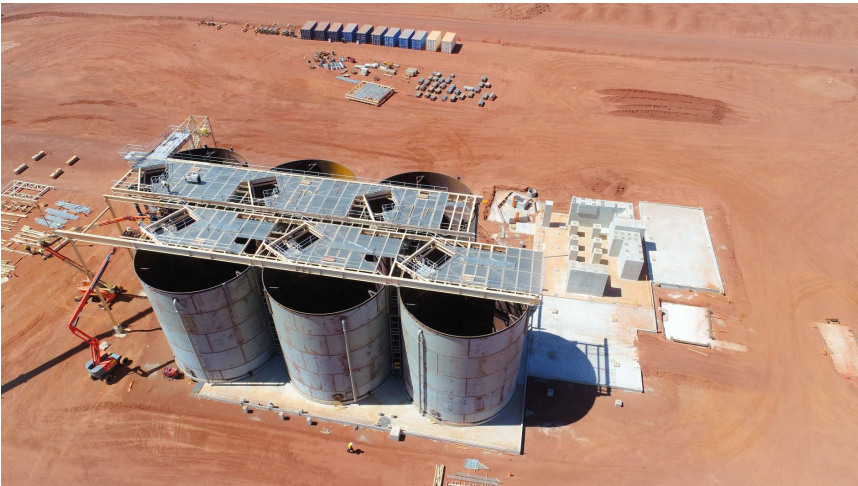
CIL tank erection
