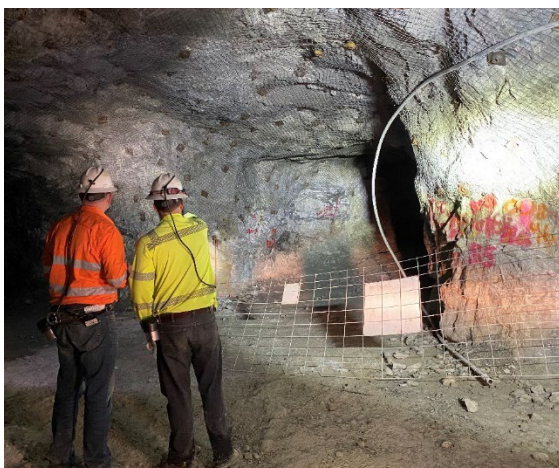
Photo 3 – Underground development drive showing good ground conditions
