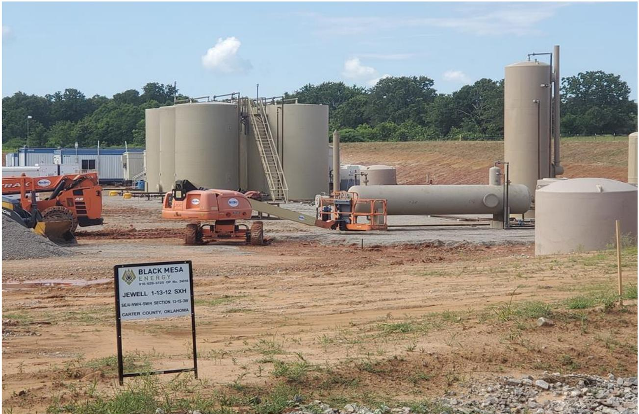
Figure 5: Jewell Well production facilities, tank battery (background) and separators (foreground).
