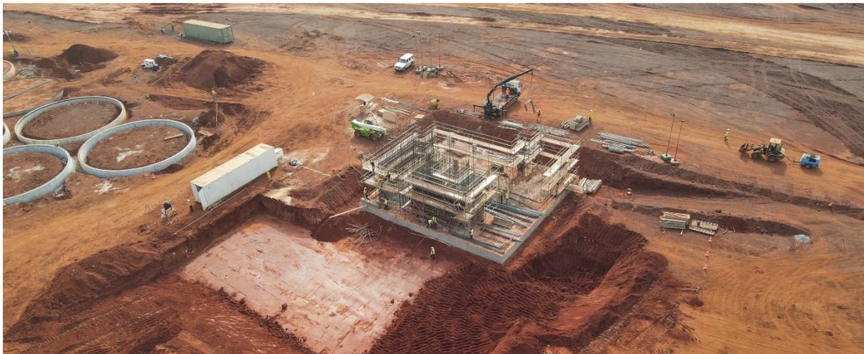
*Figure 2: Aerial view showing SAG mill raft construction*
