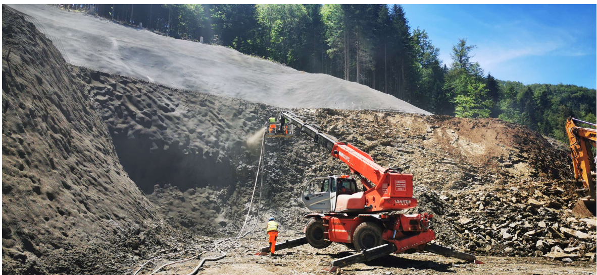
Shotcreting of the lower portal in preparation for decline construction to start
