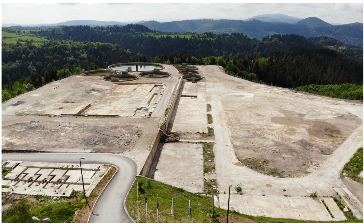
Concrete pad foundations at the Vares Processing Plant site
