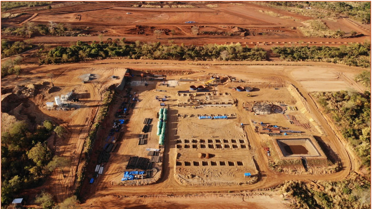
Figure 5: End of June 2022, view from the south of the processing plant area with the TSF in the background. Development of foundations for the drying, screening and packaging building can be seen in the foreground.
