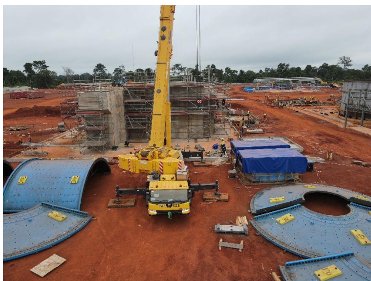
Figure 1: Overview showing construction status of Abujar's SAG Mill and CIL tanks as at 8 July 2022
