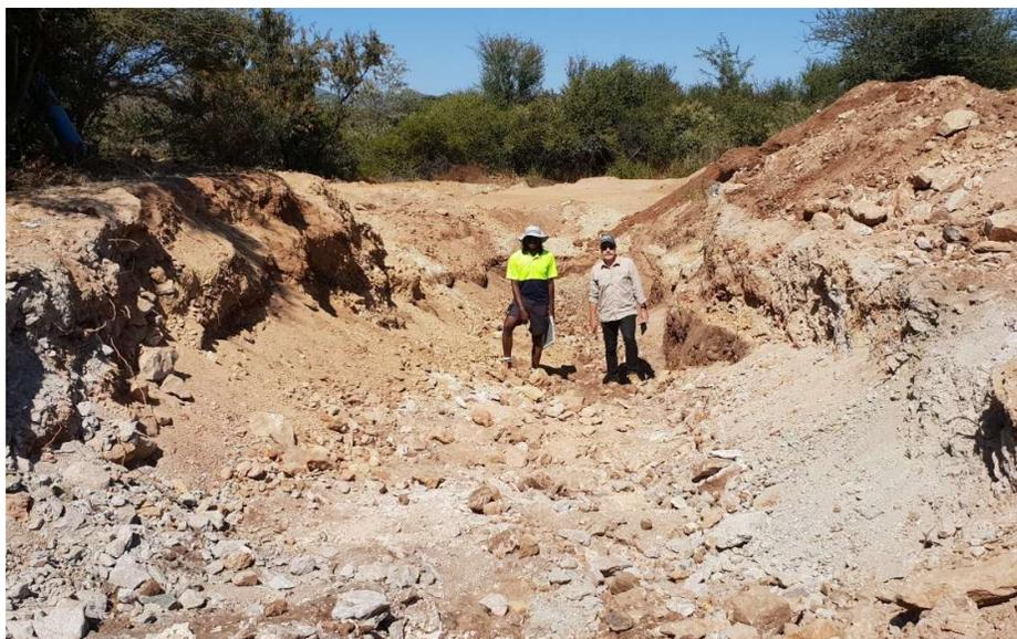
**Photo 2: Nosib Project bulk sample excavation for metallurgical testwork - with geologist, Elvis Akawa and the CEO for scale.**
