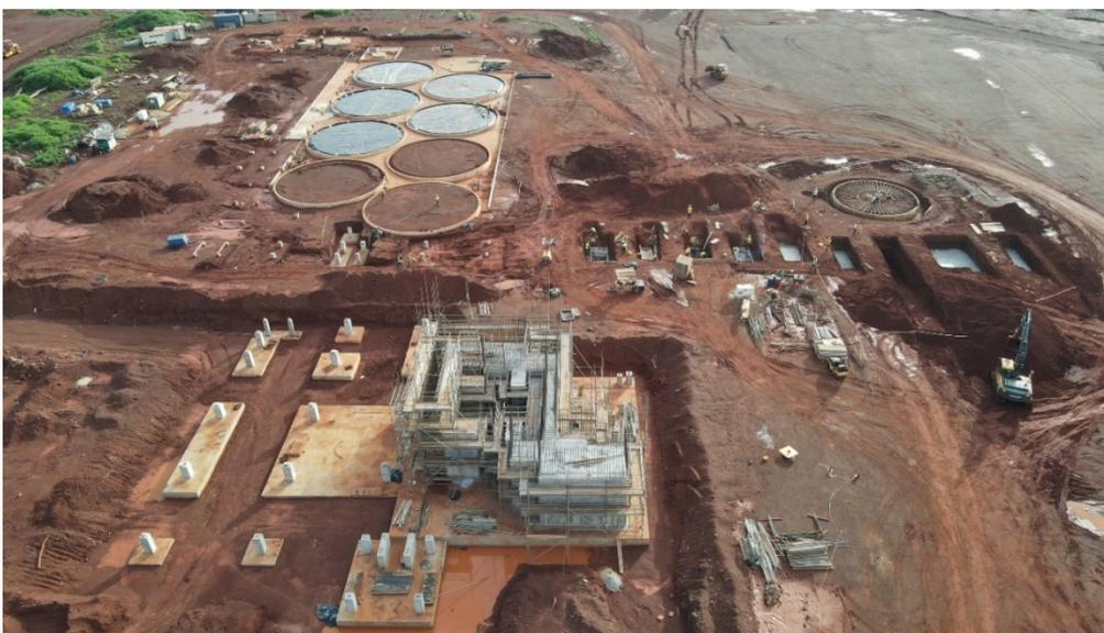
*Figure 1: Overview of Abujar Gold Project at 6<sup>th</sup> May showing location of CIL tanks and SAG Mill*
