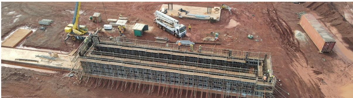
*Figure 7: Reclaim chamber wall concrete work*
