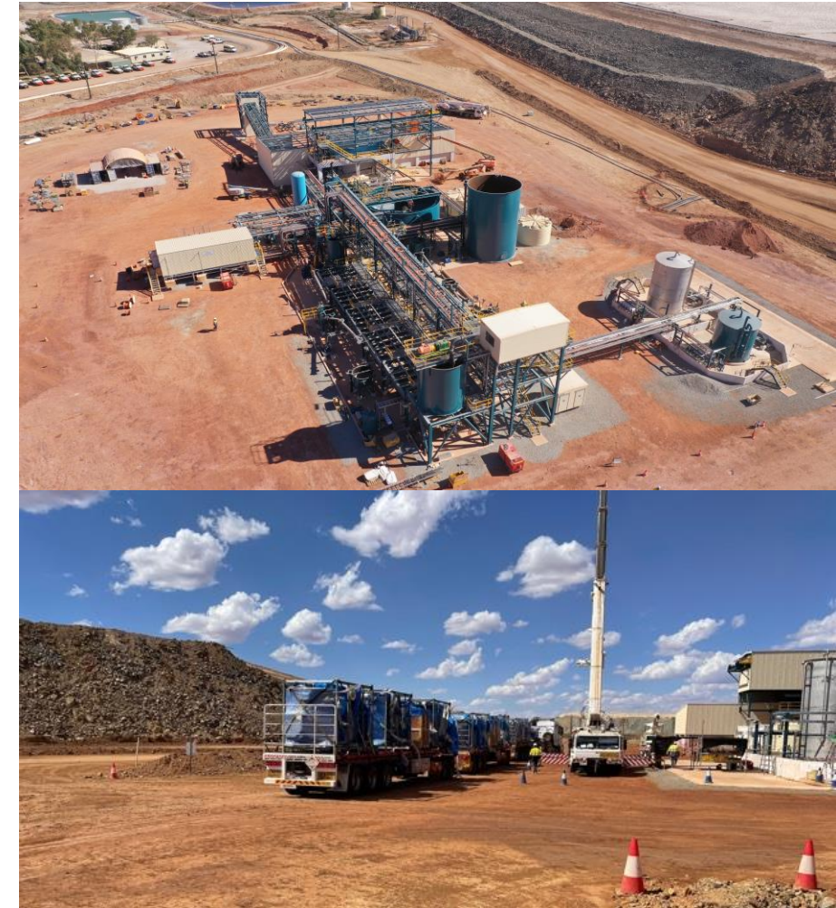
Figure 1: Concentrator at 90% Completion and Flotation Cells being Offloaded
