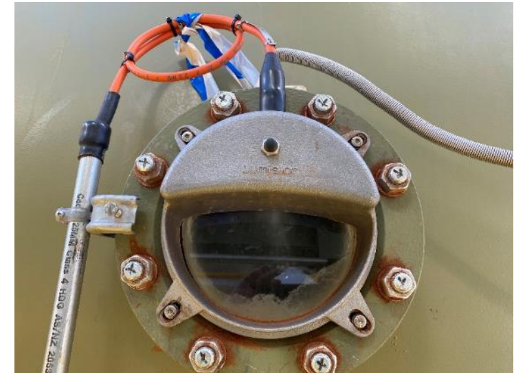
Sight Glass Showing Secondary Schoenite
