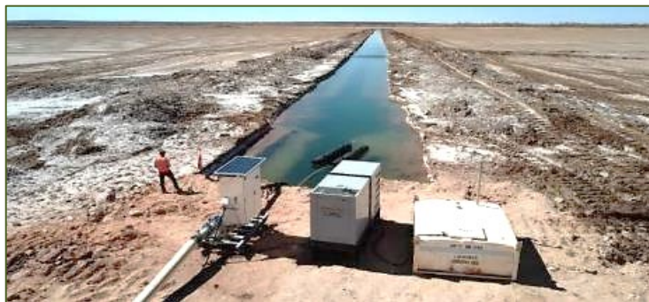
Typical Trench Pump Station
