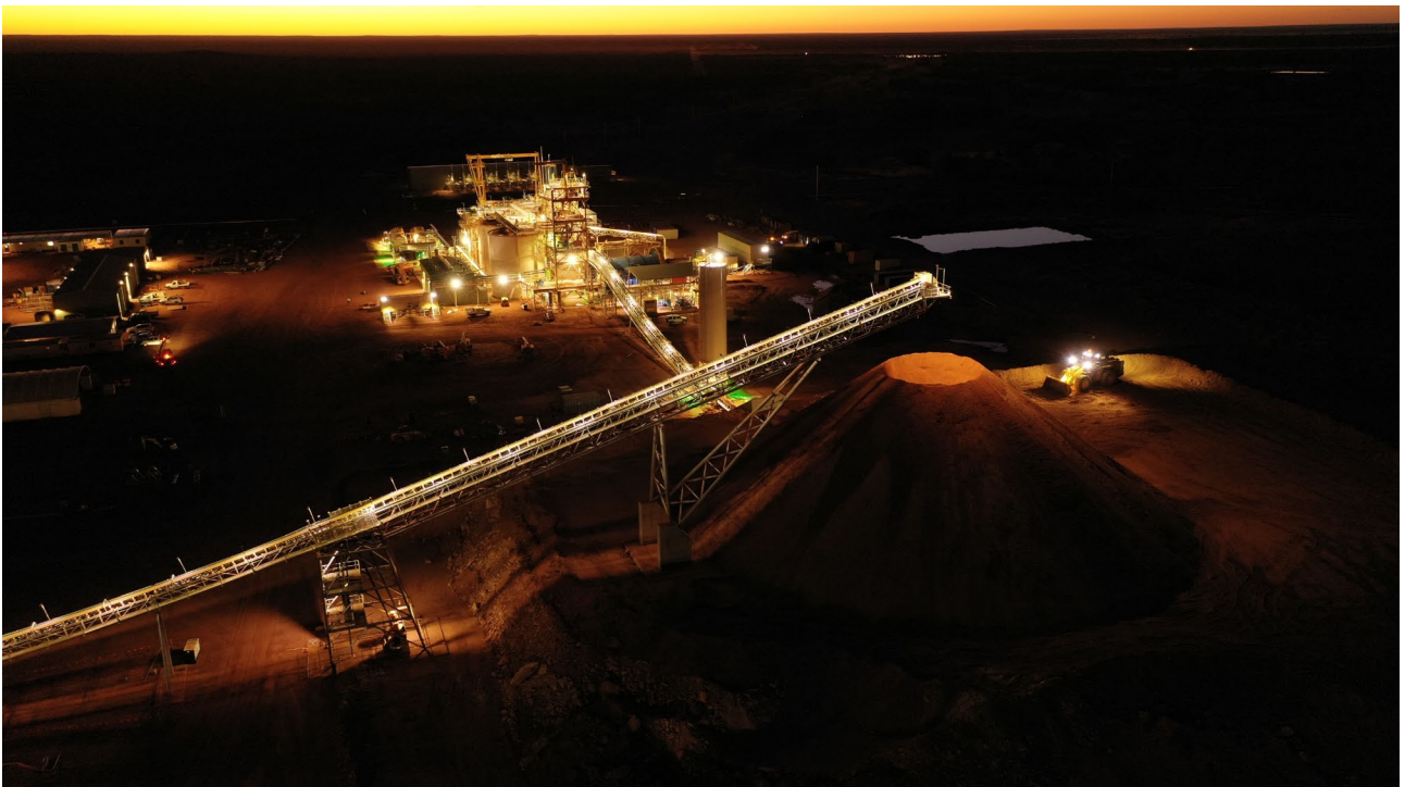
CV5 & crushed ore stockpile (foreground) and CV6, mill and CIL circuit background
