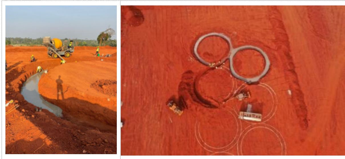
Figure 1: Blinding concrete pour for CIL Ring Beams
