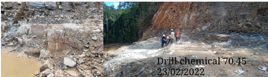
Effect of chemical rock breaking
