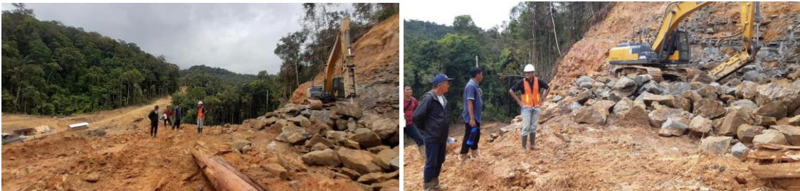
Breaking andesite with rock breaker
