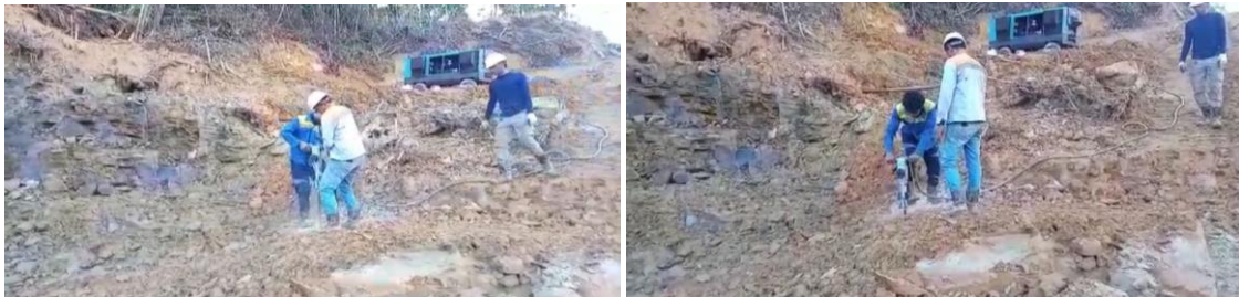
Drilling holes for chemical rock breaker
