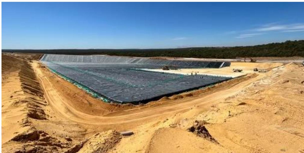
**Figure 3: Cell 1 liner installation nearing completion**
