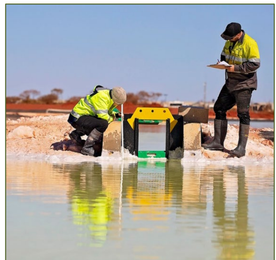
Weir Gate Adjustment
