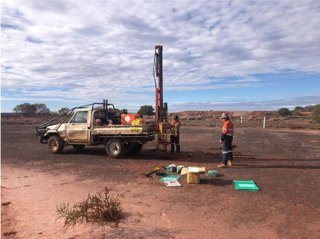
**Figure 3: Auger drilling in progress on original Horseshoe Lights gold vat**
