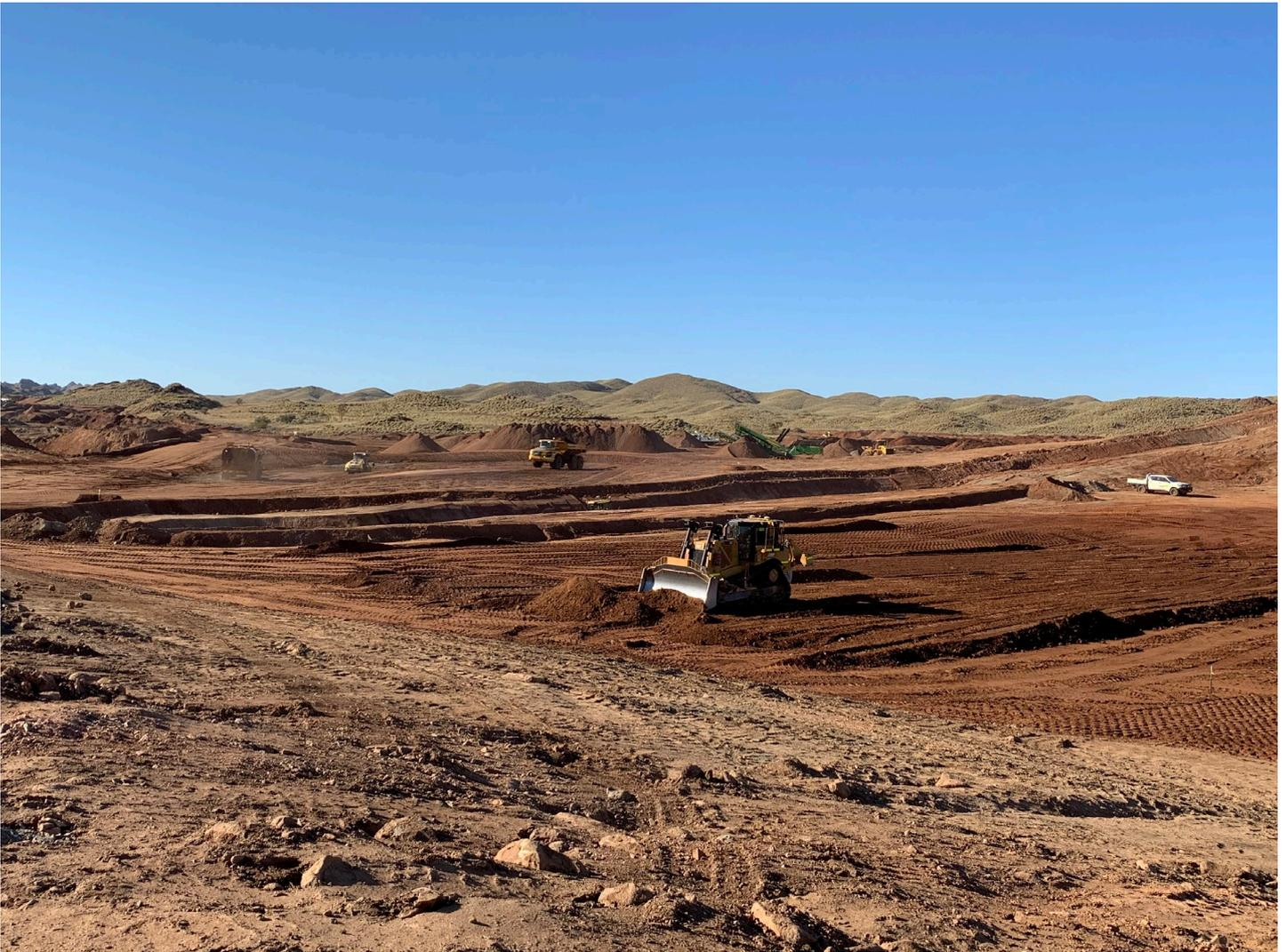
***Figure 5: Tails Dam foundation preparation***
