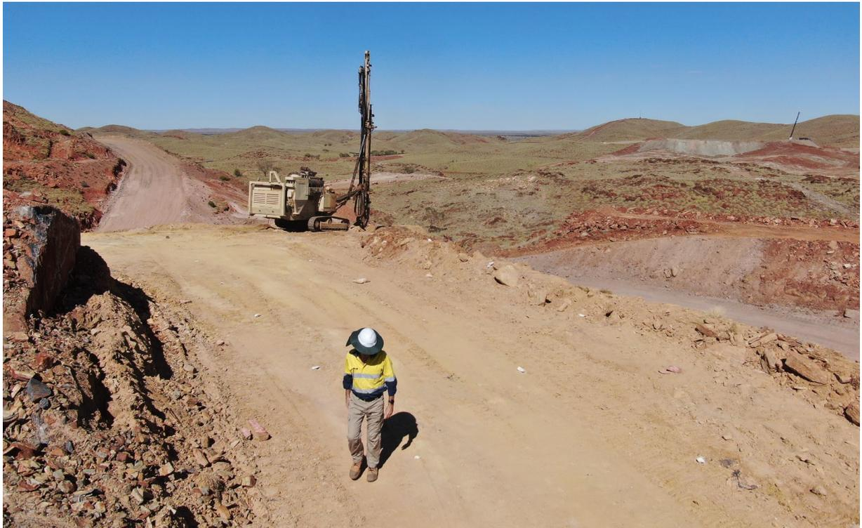
***Figure 4: Blasthole Drilling***
