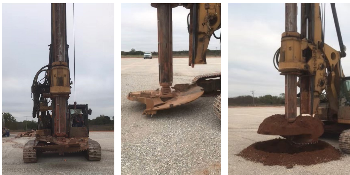
Figure 1. Drilling of the Rangers Well cellar in preparation for conductor hole drilling and casing
