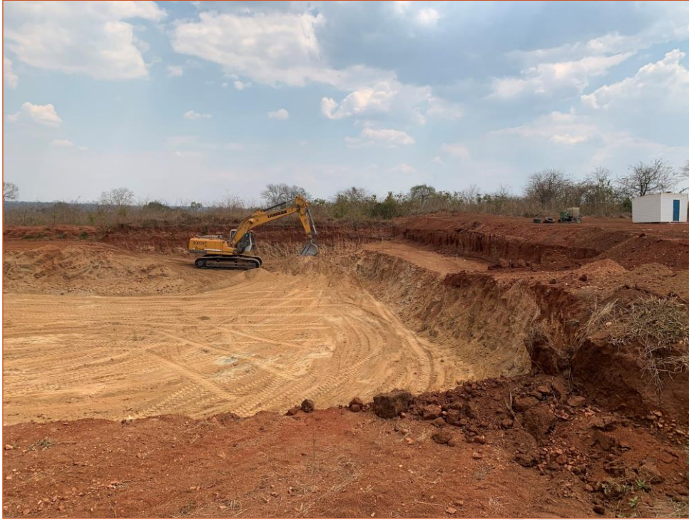
Figure 2: Terracing and levelling of the Processing Plant area.
