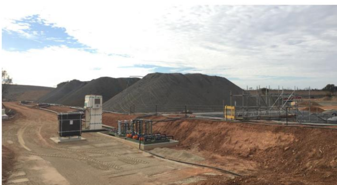
Scats Heap Leach - Heaps in the background with pump station in the foreground. PLS collection facility on the RHS
