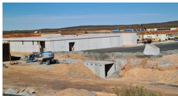
Winder house with head-frame raker leg foundation in foreground
