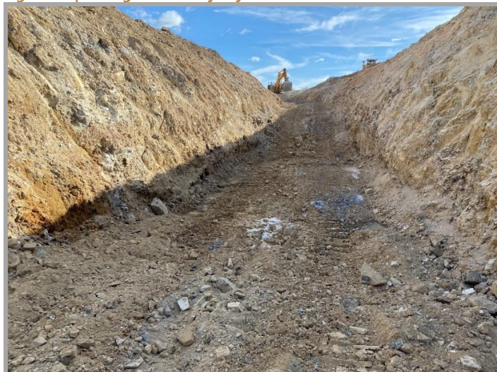
Figure 21 | Tailings Dam - Keyway Excavation works
