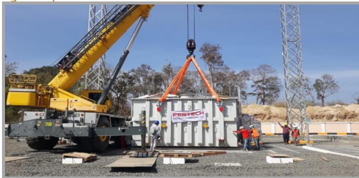
Figure 27 | Installation of Transformer
