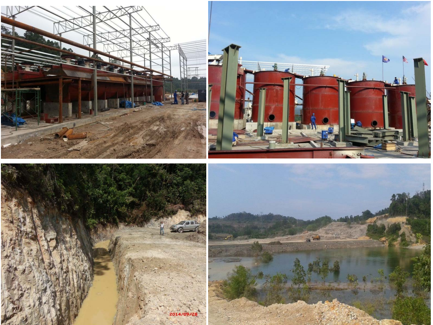
Photographs; Clockwise from top left; installation of the flotation cells and large, CIL tanks nearing completion, vista of stage 1 tailings storage facility and large run-off drain around tailings storage facility.
