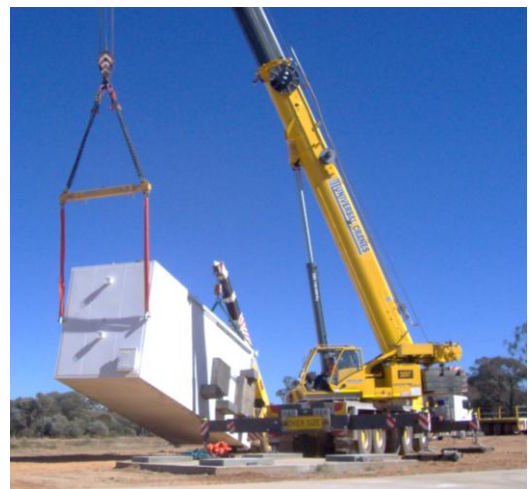
Lifting of Cold Box
