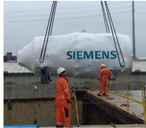
Loading of Unit 2 Turbine
